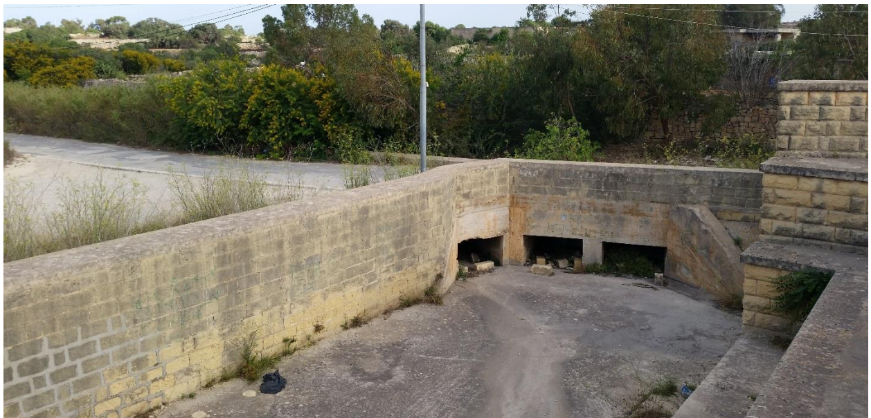
Figure 2 - Lowest part of the open reservoir complex, showing overflow culverts channelling storm water into the valley watercourse adjacent to the site
