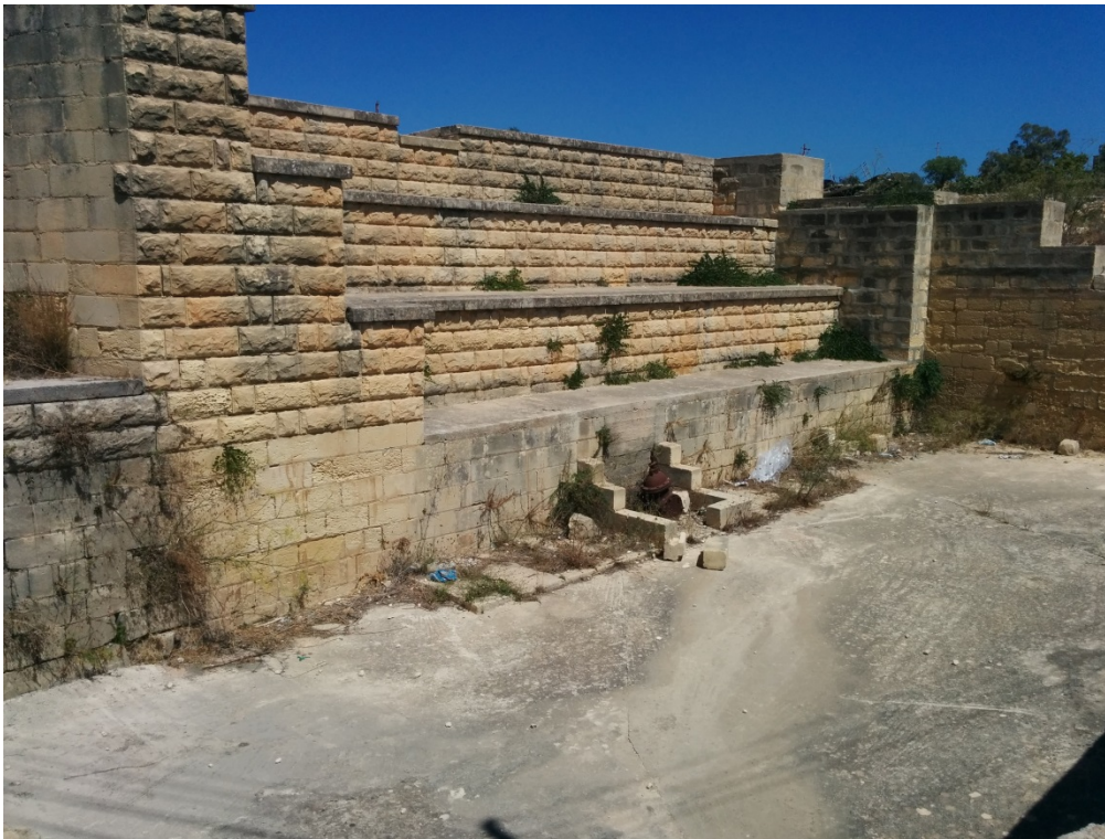
Plate 4: Retaining wall at downstream end of the Has-Saptan infiltration basin, showing outlet valve at base.
