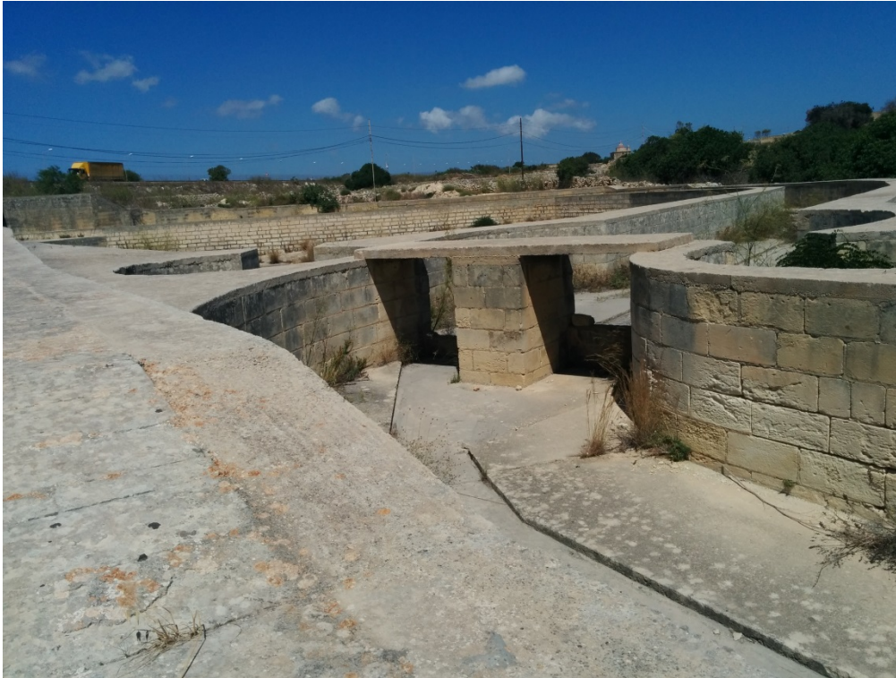
Plate 3: Internal view of Has-Saptan infiltration basin showing minimal depth of 4 courses (1m)
