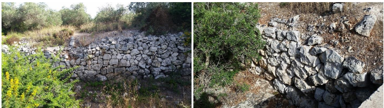
Figure 11 - rubble wall containing fill, adjacent to watercourse
