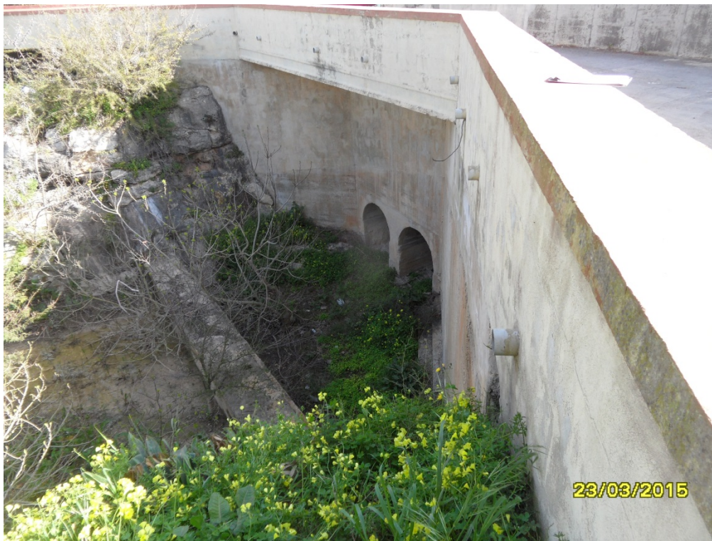
Plate 6: Pair of discharge outlets from dam/bridge on Wied Has-Saptan downstream of existing facility.
