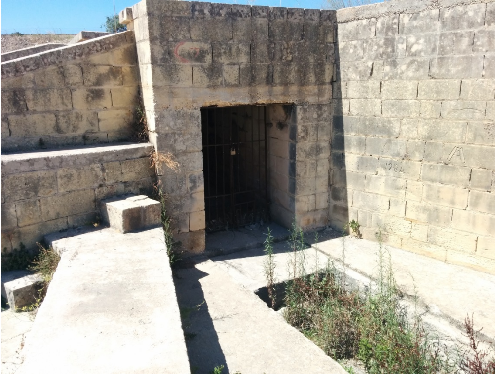
Plate 2: Inlet to Has-Saptan infiltration basin from Malta international Airport main runway
