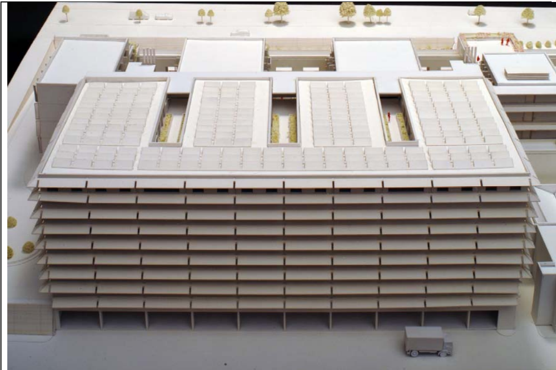
PLATE 7 CAR PARK SOUTH FAÇADE (PHOTOVOLTAICS ON THE ROOF & ON LOUVRES)
